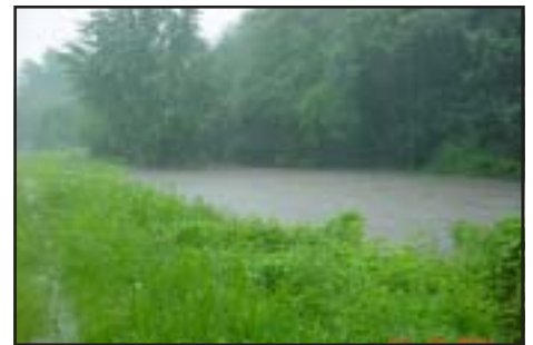
The first big test! Only one month after completion, the stream overflows its banks completely covering the weir. It went on to survive another bankfull event and two hurricanes. The only damage after a harsh summer was two fallen stones easily restored with the loader.
