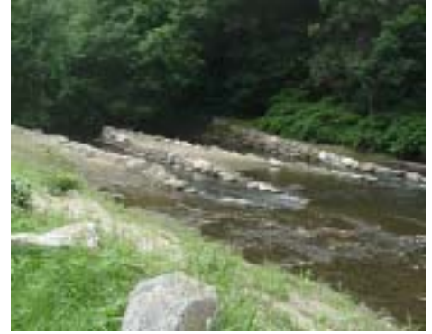
Once the second arm was completed all erosion controls were removed and the banks received a final grade. The stream flowed freely through the two points and began to scour out holes in the channel as designed. Coir matting was placed on disturbed banks and native plants, seeds and live stakes were installed. This picture shows the weir completed and functioning.
