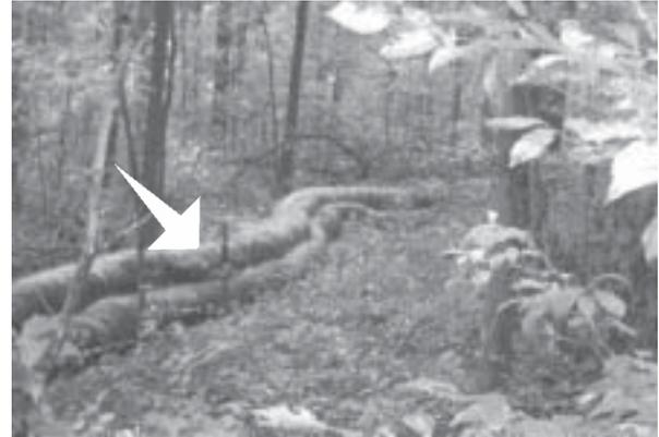
To use this BMP for a submittal, the silt fence slope limitations are acceptable. The Soxs are installed on the contour and can function as a silt fence replacement and or as filter berms. Soxs utilize their weight and stakes for reinforcement. Soxs can also be installed in forested areas with little or no disturbance. The mulch medium is blown into the Soxs. Once the project is completed, the Soxs are cut open and the material spread in place as mulch.
