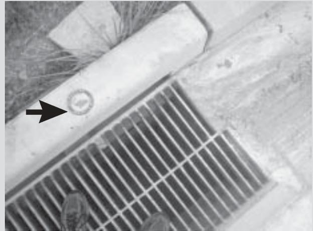
I took this photo at a site in East Fallowfield. Note the stamp on the curb. The material going into the inlet is from a concrete washout. The weather was dry as a bone, which makes this even more moronic. Enjoy.
