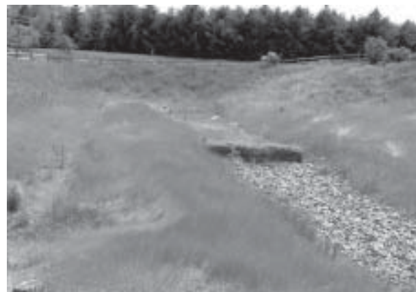
After: Elevated berm extends flow path in basin and provides greater recharge capabilities. The sediment forebay filters stormwater before it discharges from the basin.
