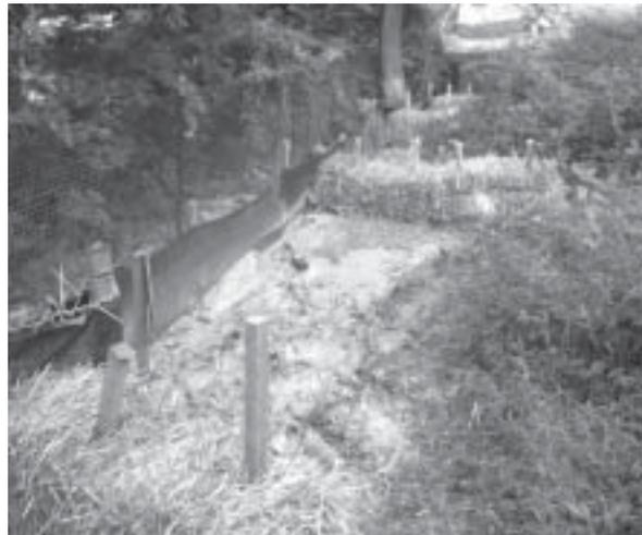
*Silt fence installed down a hill, hay bales added to try to check flow, and failing rock filter at bottom of hill*
