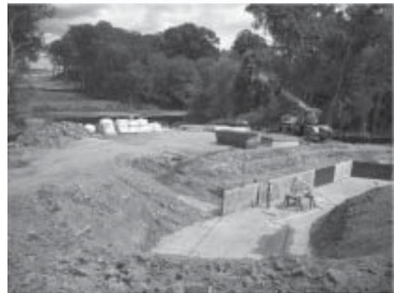
*Western abutment foundation under construction in August 2010, for the four-span 202 Parkway bridge over the Neshaminy Creek. Super silt fence has been installed on both sides of the Neshaminy along with "jersey barriers" and a sand bag cofferdam.*
