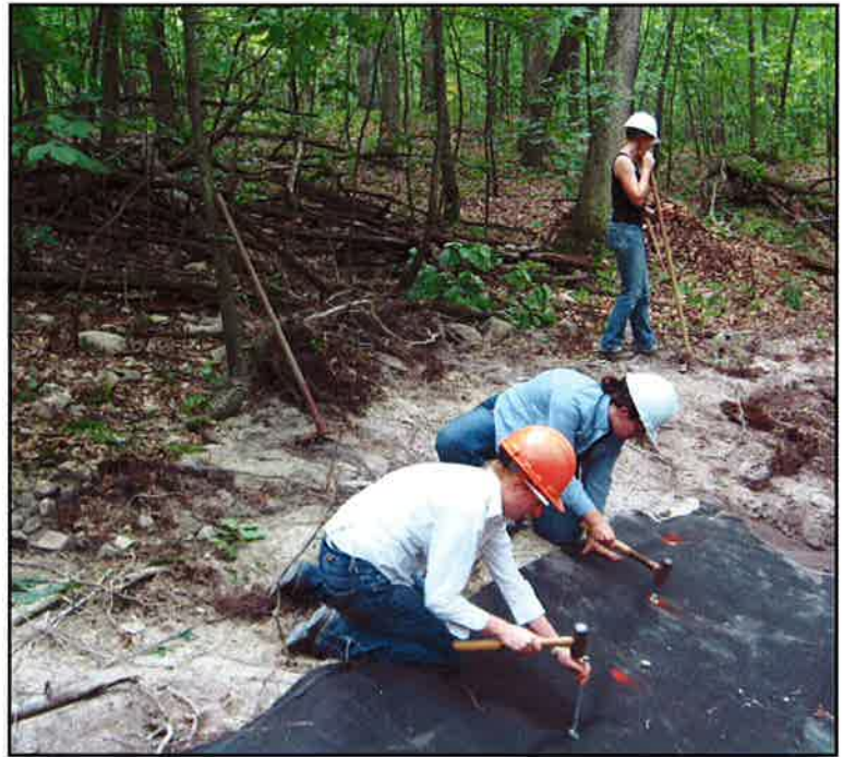
Rachel Onuska and Meghan Rogalus work to secure a vernal pond liner at the wetland restoration workshop at Kings Gap State Park.
