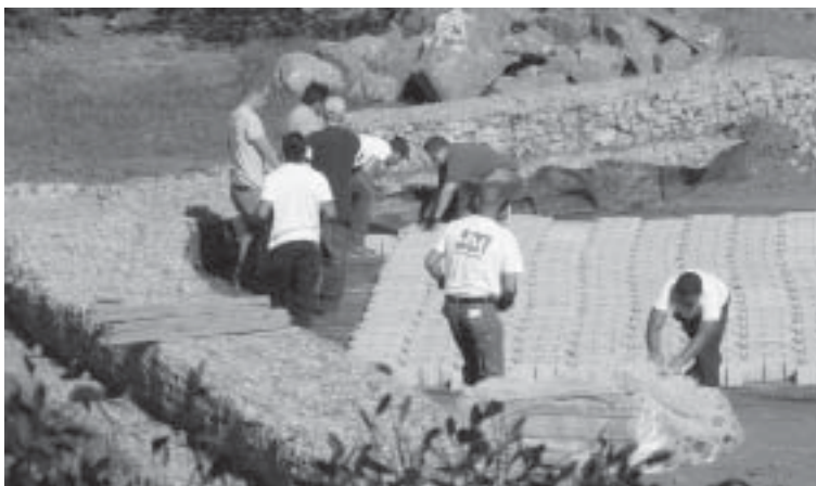
Volunteers installing concrete blocks in forebay during a two-day work event.
