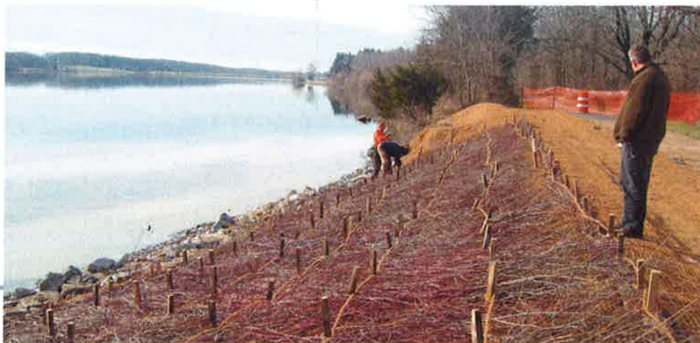
Eric Wightman observes workers as they place live stakes during construction.
