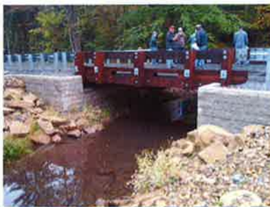
Officials tour one of the new dirt and gravel roads after completion.
